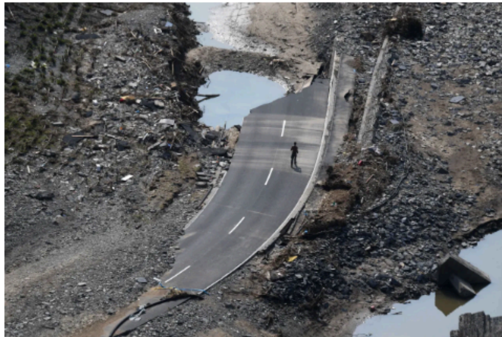
A person walks along a section of highway near Mayschoss, Germany, that was damaged from heavy rains and flooding, in mid-July. Photograph by Christof Stache / AFP / Getty
